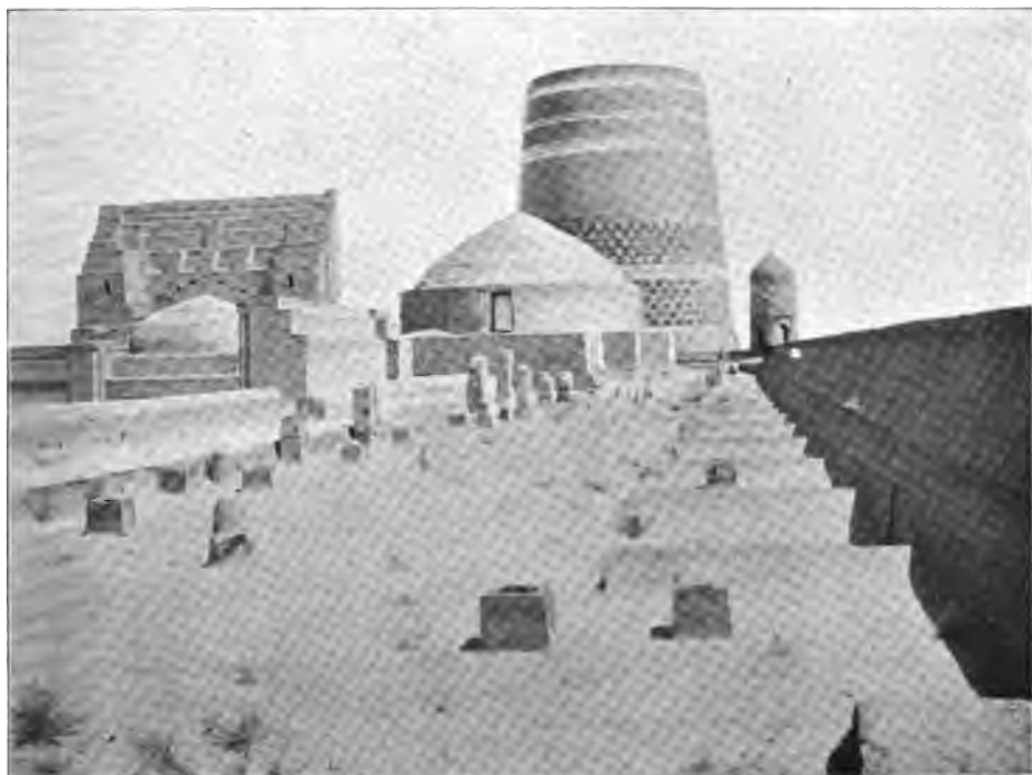
Outlook across the roof on the medrese of Mahommad Amin Bahadur Khan in the town of Khiva.
