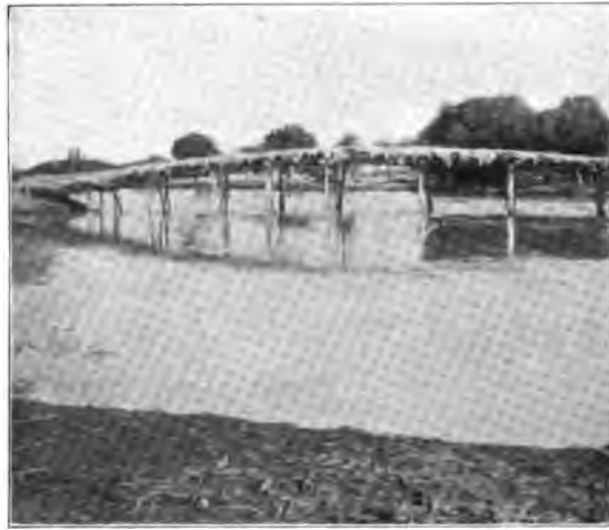
Bridge across the canal from the Amu Darya to Khiva.
