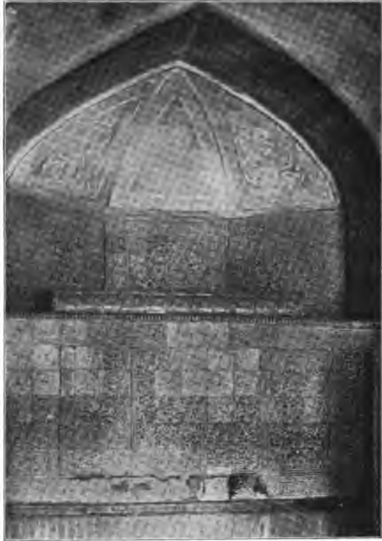
Ibrahim Khosha's sepulchral chamber at Khiva. In the foreground the rectangular kabr covered with majolica; the upper part is pointed. The niche in the sepulchral chamber is like the sarcophagus covered with splendid majolica in white and blue designs.
