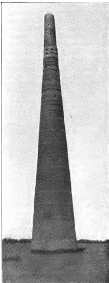
The minaret of Sultan Mahomed Karashmishah near Kona Urgendtsh.
